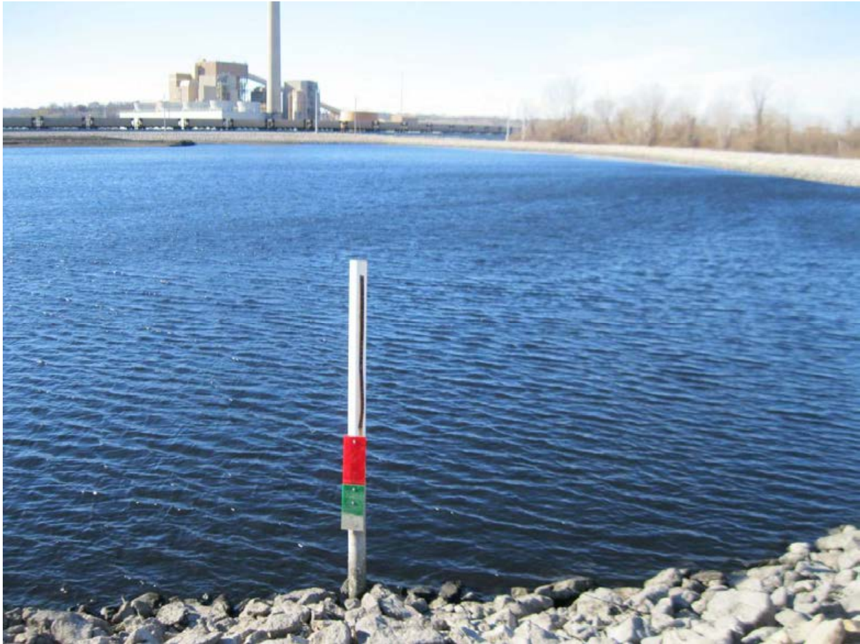
Figure 3-1 Water Level Indicator
