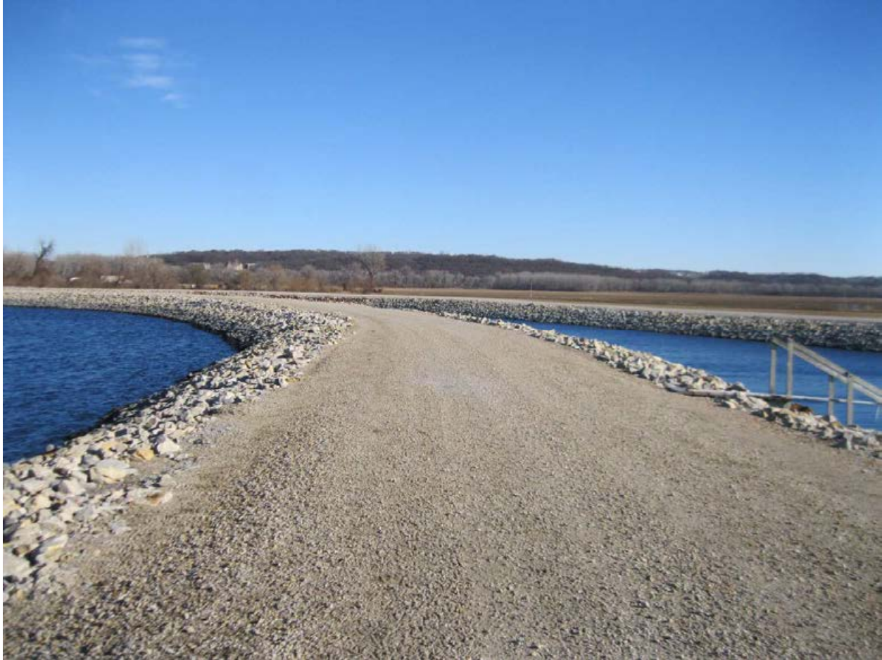
Figure 4-1 Interior Dike Crest Condition
