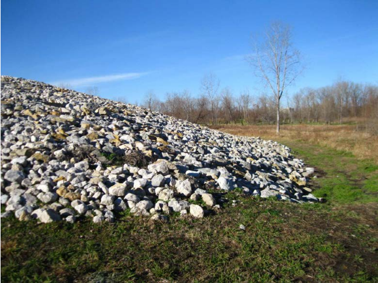
Figure 4-5 Exterior Dike Recent Riprap Placement.
