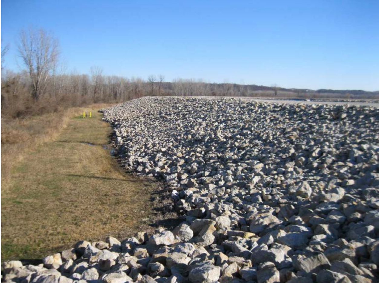
Figure 4-3 Exterior Dike Slope in North Facing Slope of Impoundment
